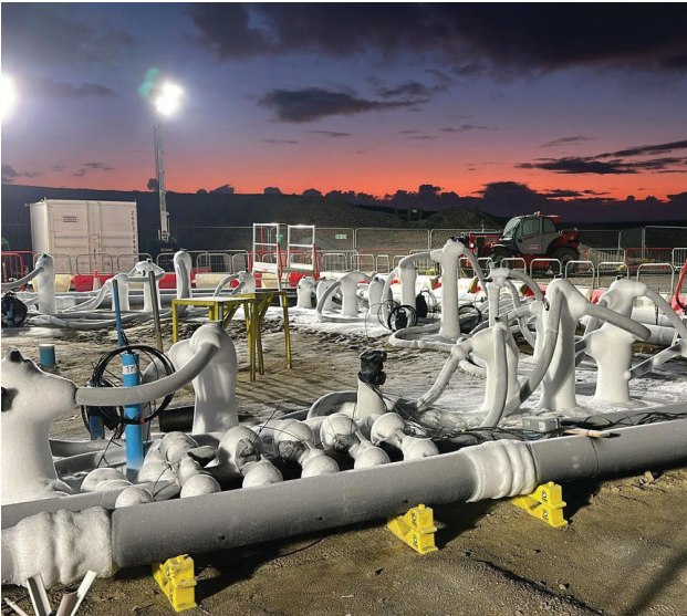
Sizewell C Ground Freezing Trial
