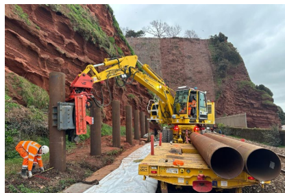
Specialist Piling and Rail
